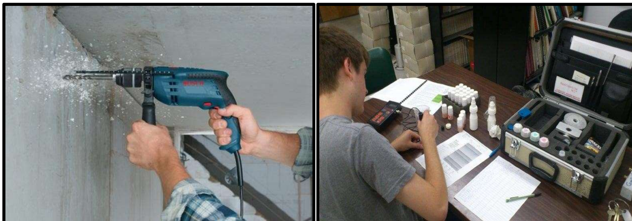
(a) Drilling of concrete element
